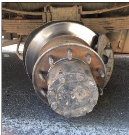
Rotor resting on pavement. Notice bent studs on the left.
